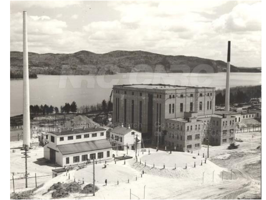
NRX and Zeep buildings, Chalk River Laboratories, 1945
