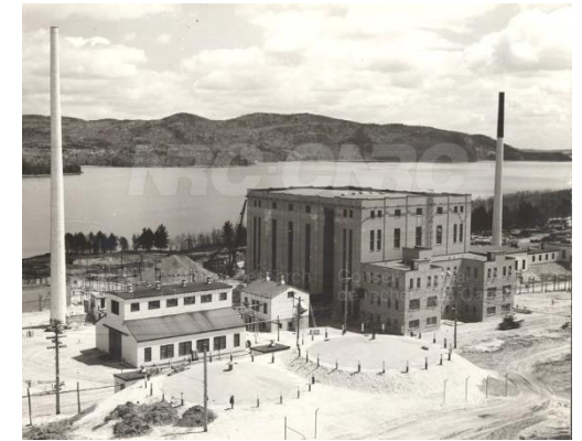
NRX and Zeep buildings, Chalk River Laboratories, 1945
