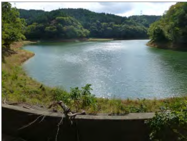
Ogi dam lake, Kawauchi
