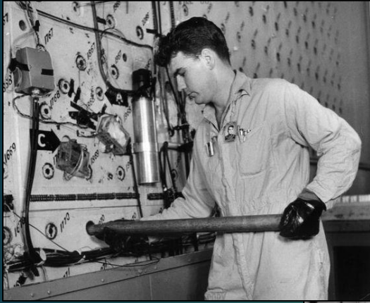
U cores into reactor
